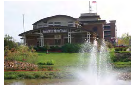
A parking deck or ramp may be needed in the future to accommodate increased demand for the Northstar commuter rail.
