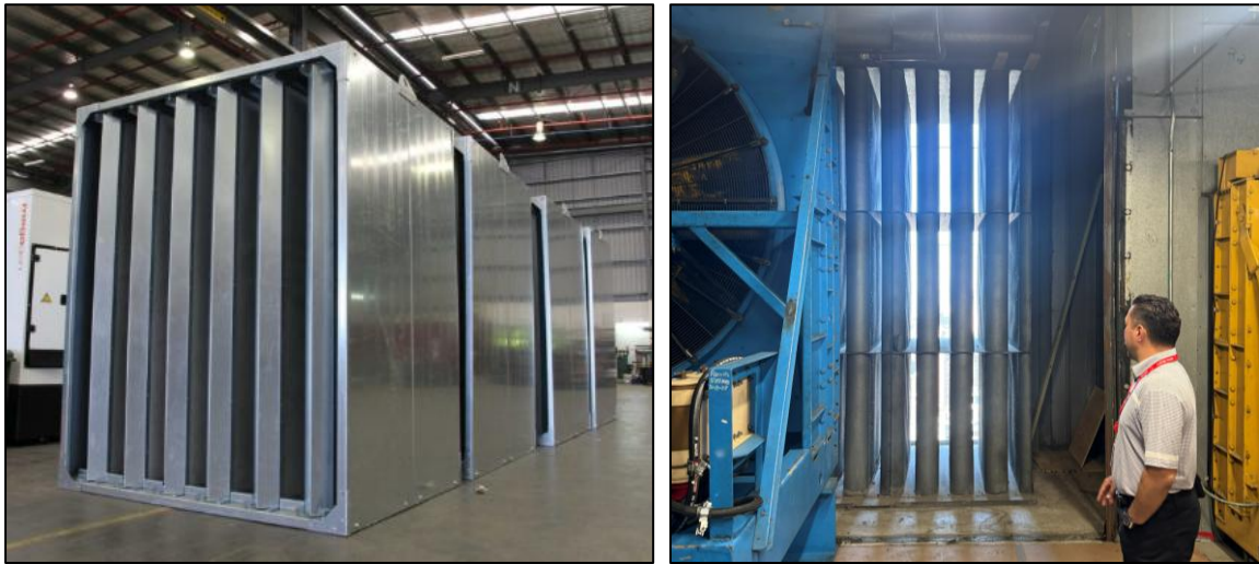
Figure D-6: Commercial Acoustics photos showing generator noise control silencers.
