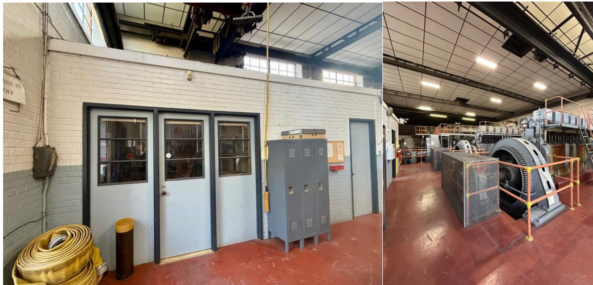
(Left) 1947 Diesel Engine. Image by LEO A DALY on October 11, 2024. (Right) Brick interior partitions. Image by LEO A DALY on October 11, 2024.
