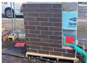
Pre-Cast Wall Panel Mock-Ups
